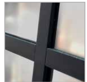
glazing bars glued onto the glass
