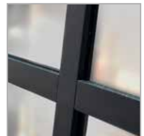
glazing bars glued onto the glass
