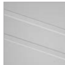
milling on the surface of the door leaf, width 15 mm in version B12
