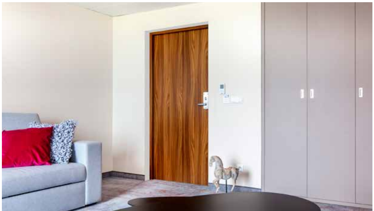
G46 door, fixed wooden door frame
